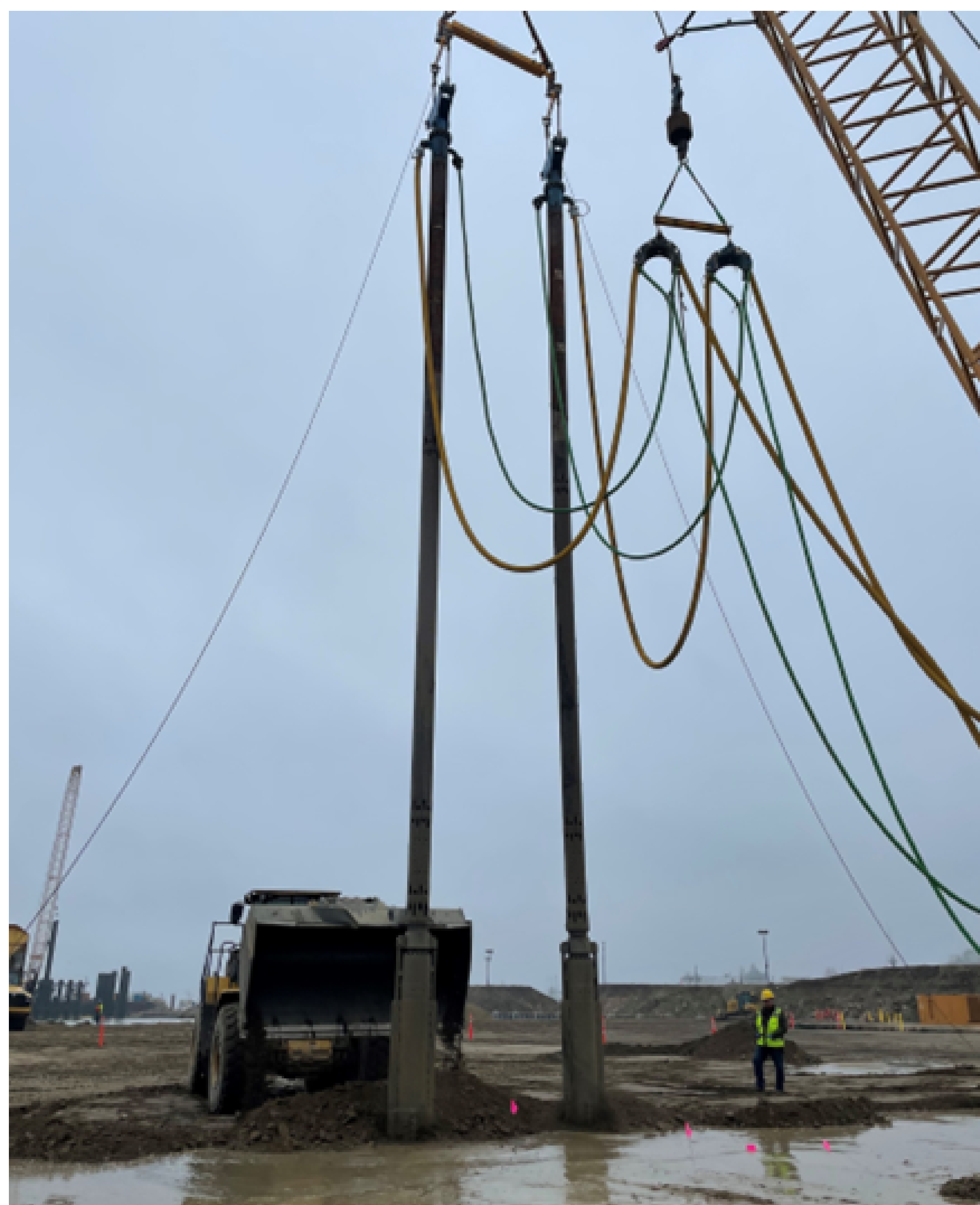
Tandem Vibrocompaction Rig - First in U.S.
