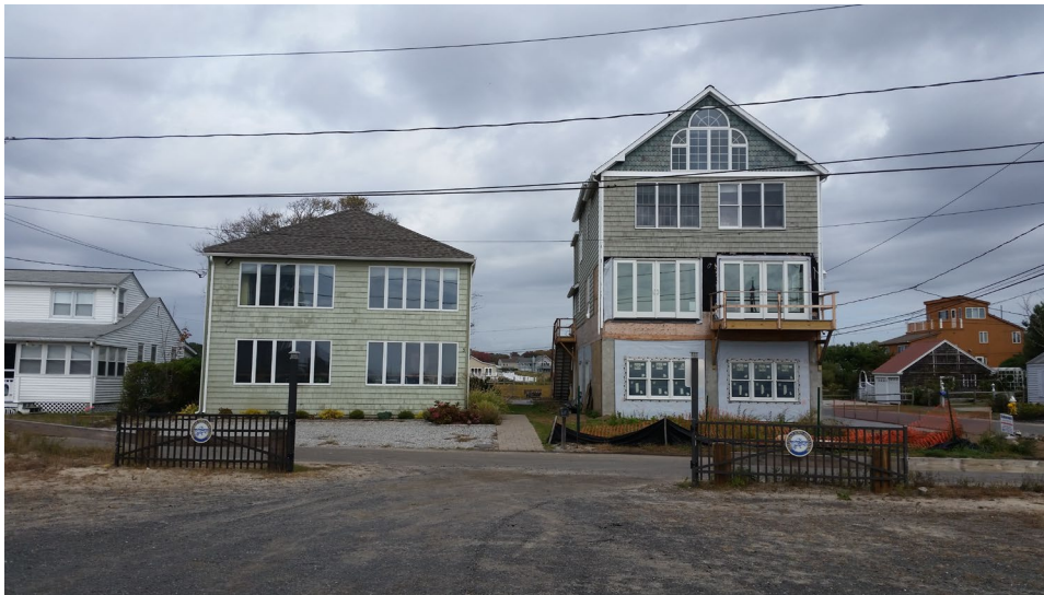
Figure 4. Two houses in the coastal municipality of Old Saybrook, Connecticut. The house on the right is in the process of being elevated. 156
