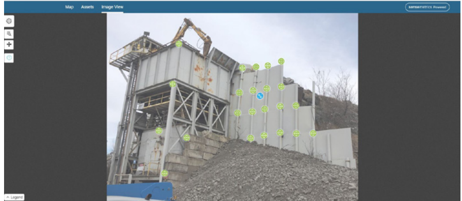
Image view on Sensemetrics Software Platform of retaining wall structure being remotely monitored.
