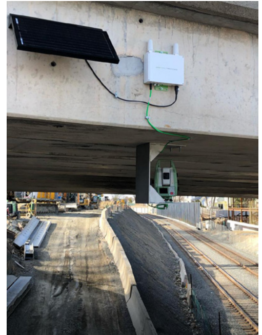
Robotic Total Station providing real-time survey data of adjacent tracks.
