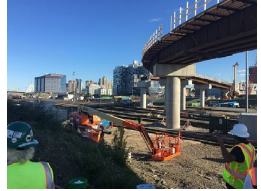
The CI Boston Chapter visits the Green Line Extension Project in September
