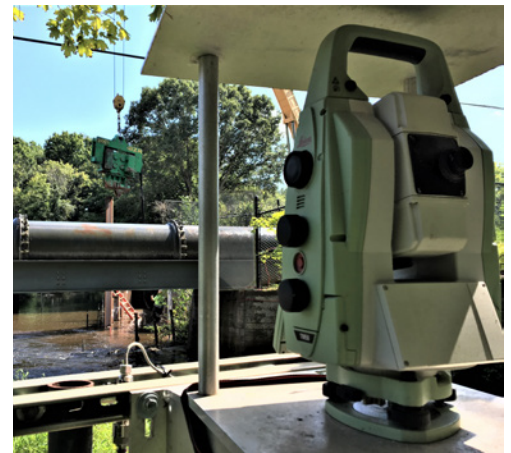
Robotic Total Station, Tiltmeters, and Seismographs monitoring critical utility infrastructure during sheet pile installation.
