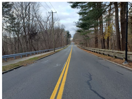
View of top of dam on Armory Street with trees requiring removal along dam slopes
