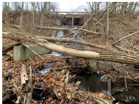
Spillway chute that needs replacement with fallen trees
